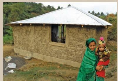
Straws bales are stacked on a gravel foundation; a door and a roof are added; and the house is ready to be covered in plaster.
