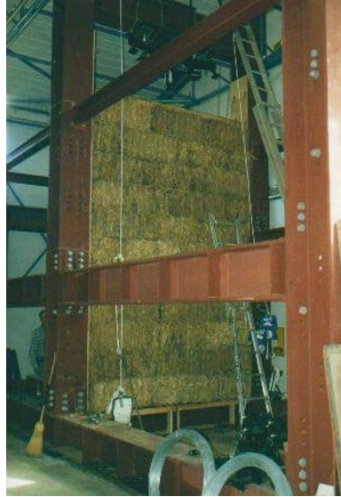
Figure 1 General view of steel test frame and partly completed wall (Photograph: P. Florence)
