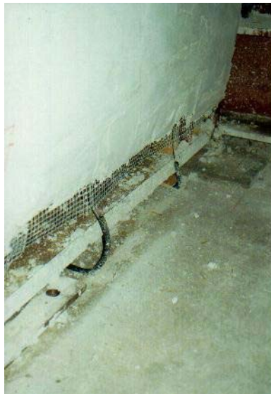
Figure 14. View of bottom plate after test (Photograph P. Florence)
