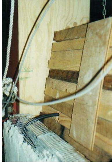
Figure 15. View of top plate after the test. (Photograph P. Florence)
