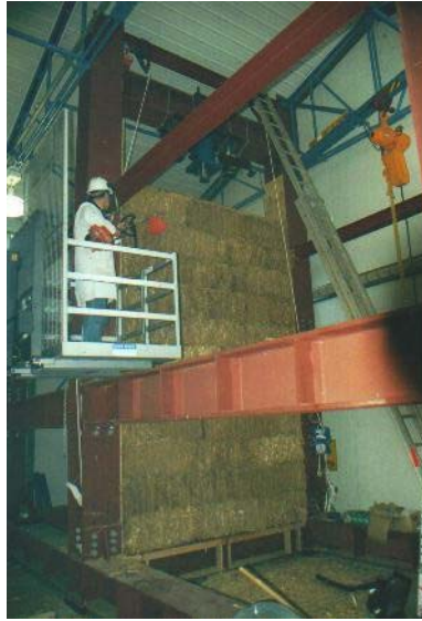
Figure 4: Trimming wall to size. (Photograph P. Florence)
