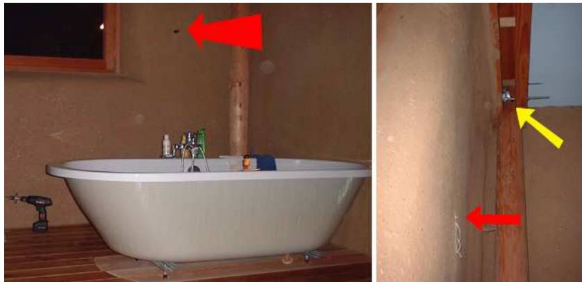
Figure 4.23: Monitors #1,2, and 3 fit into one channel that was drilled across the earth plastered exterior straw bale wall in bathroom of the family house in Blanden (see the red arrows). On the right , there is a view along the wall towards the ceiling. Monitor #4 was placed directly under the ceiling (see the yellow arrow).
