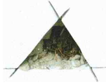
Figure 4.6: A wall opened under the corner of the window sill without a drip edge reveals musty smelling, weak, moist straw. From Platts (1997).
