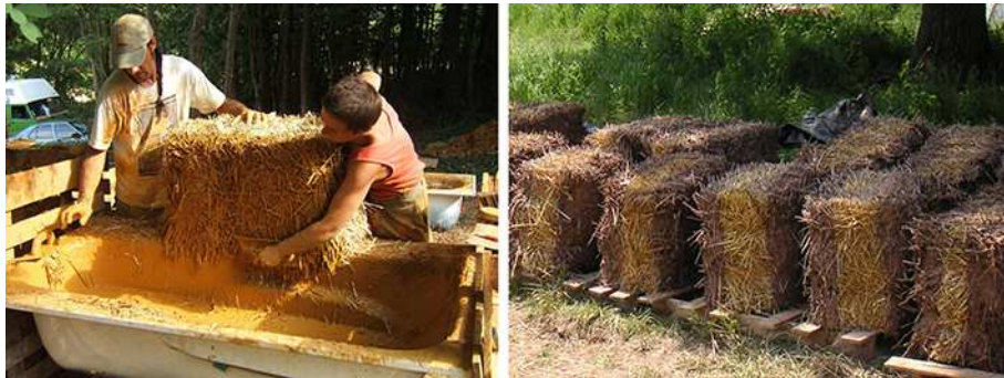
Figure 7.7: Prior to being placed in the wall, straw bales are dipped on their exterior and interior facing sides in a water-rich clay solution (clay slip) and stored on pallets to dry a bit. Photography by Tom Rijven.
