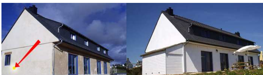
Figure 4.19: Straw bale house in Plozevet, Brittany, France. On the left —February 2006—The red arrow points at the approximate position of the monitor in the western wall. At the time of the storm, the monitored bale was approximately 400 mm above the ground (see fig. 4.14). On the right —July 2006—Since March 2006, the lime plastered house has been further protected from frequent storms by timber cladding. A storage shed was built at the place of the greatest damage. The shed created a space allowing for ventilation so that the wall covered by it could dry out more easily. At the same time, the shed and the timber cladding (although ventilated) prevented drying, which could have been considerably improved during spring and summer due to sun and wind exposure.
