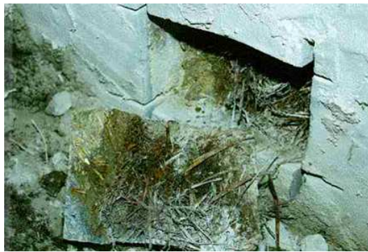
Figure 4.5: ”White mould indicates advanced rotting of supersaturated straw - moisture content off scale. 1m above this location, straw was moist and deteriorating with measured moisture content about 38-43%” (presumably dry-weight basis - ed. author). From Platts (1997).
