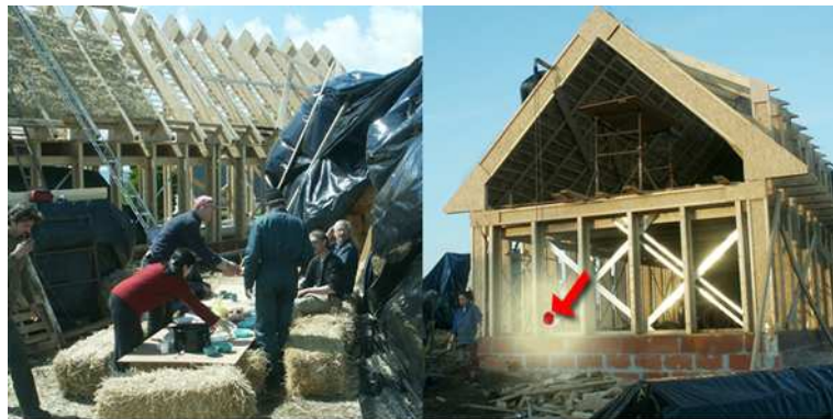
Figure 4.14: Straw bales on the edge are used in the walls as well as in the roof. The red arrow points at the future location of the monitor. Photography by Martin Oehlmann.
