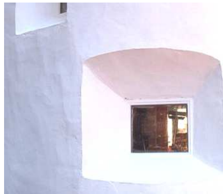
Figure 4.7: No drip edge on the window sill is a bad practice in straw bale construction. Photo of lime plastered straw bale house in Maine, USA by Beals (2004).
